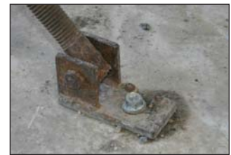
The Titen HD 3/4 x 6 and 3/4 x 7 have a 1" section under the head that is unthreaded to allow installation into tilt-up wall braces.
